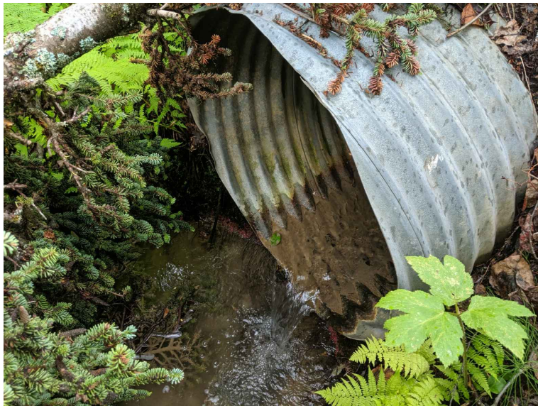
Existing Culvert Outlet
