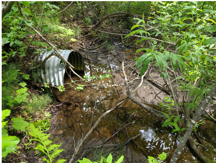
Existing Culvert Inlet
